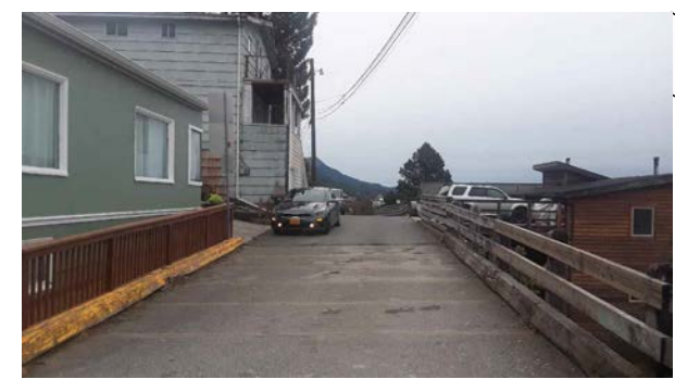
LOOKING SE, UPSTATION, SAYLES ST.
