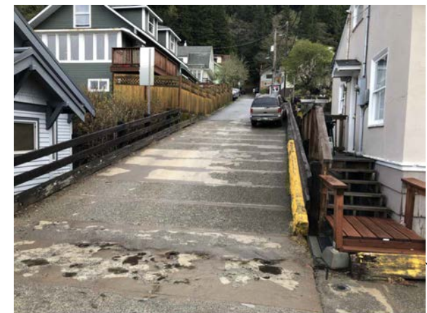
LOOKING NE, DOWNSTATION, GORGE ST.
